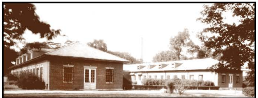
Work buildings on the grounds of Columbus State Institute were converted from dormitory cottages.
