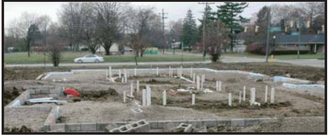
Meanwhile work is continuing at the South James and Scottwood location.
